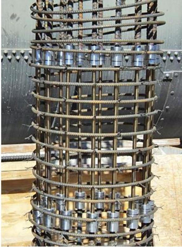
Figure 70. Construction of the Pier using Superelastic SMA and ECC as structural elements in the Plastic Hinge, Seattle, U.S.A. Source: (Clines, 2017).
