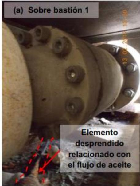
Figure 30. State of the shock-transmitters of the Bridge on bastions with dust, moisture, and trash inside the cover. Source: (Vargas-Alas et al., 2017)
