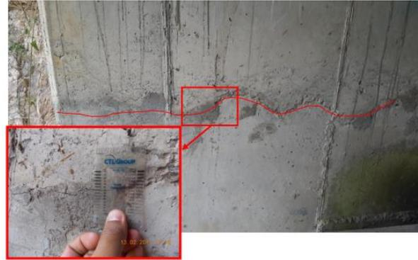
Figure 32. Cracks in the bastions of the Salitral Bridge. Source: (Vargas-Alas et al., 2017)
