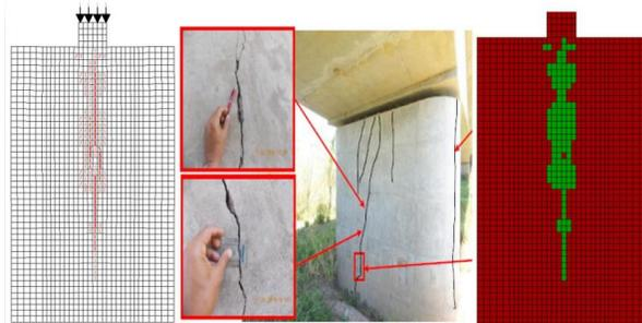
Figure 75. Comparison between the cracked pier and the analytical Model with concentrated axial.
