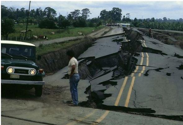
Figure 16. Consequences of 1991 Earthquake in Limon, Costa Rica.
