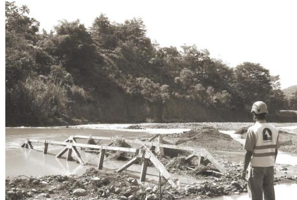
Figure 21. Truss of the Bridge over the Pacuare River in National Route N° 243 that collapse as a consequence of the Tropical Storm Nate, Costa Rica 2017.
