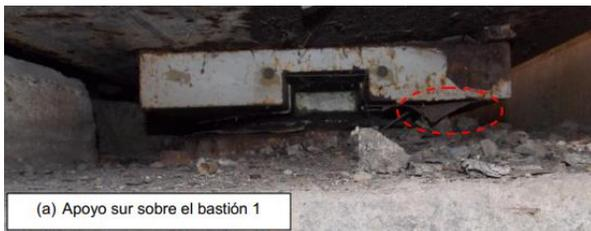
Figure 31. Detachment of the paint and corrosion protection system, PTFE pot bearing, support south of Bastion 1. Source: (Vargas-Alas et al., 2017)
