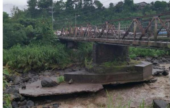
Figure 35. Affectation of the foundation of the pier of the Bridge "La Alegria" caused by the effects of the river, Turrialba, Costa Rica (2015).
