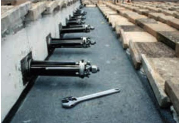
Figure 60. SMADs as installed in the Basilica of San Francesco in Assisi, Italy. Source: (FIP, 2016)
