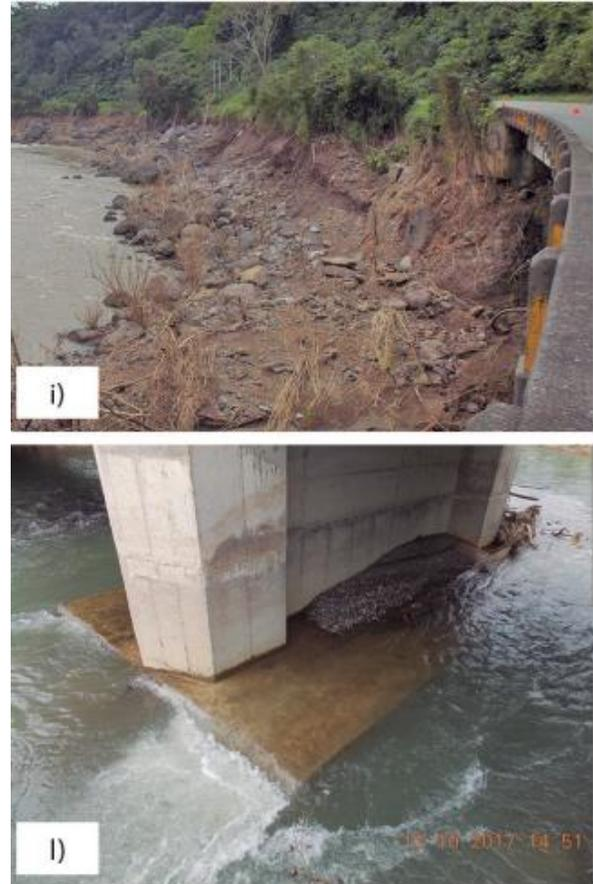
Figure 19. Damages in the Bridges of Costa Rica as a consequence of NATE Storm, Universidad de Costa Rica. Source: (Muñoz-Barrantes, 2017)
