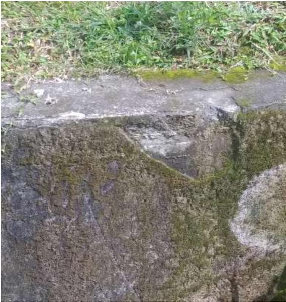
A photograph of a concrete curb. The top surface of the curb is severely damaged, showing large areas of delamination where the concrete has chipped away, revealing a rough, porous interior. There is significant moss and algae growth on the damaged surface and the adjacent ground.                |
