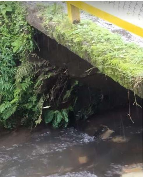
A photograph showing a concrete structure, likely a bastión or retaining wall, that has suffered from significant erosion. The structure is partially submerged in water, and there is a large amount of green vegetation growing on and around it. The water is dark and turbulent, indicating a strong flow. |
