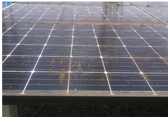
Fig. 2. Soiled PV module.
