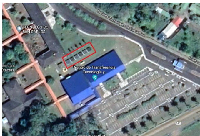
Fig. 5. Aerial photograph of TEC's photovoltaic station (identified in red) located in San Carlos. Source: Google Maps.
