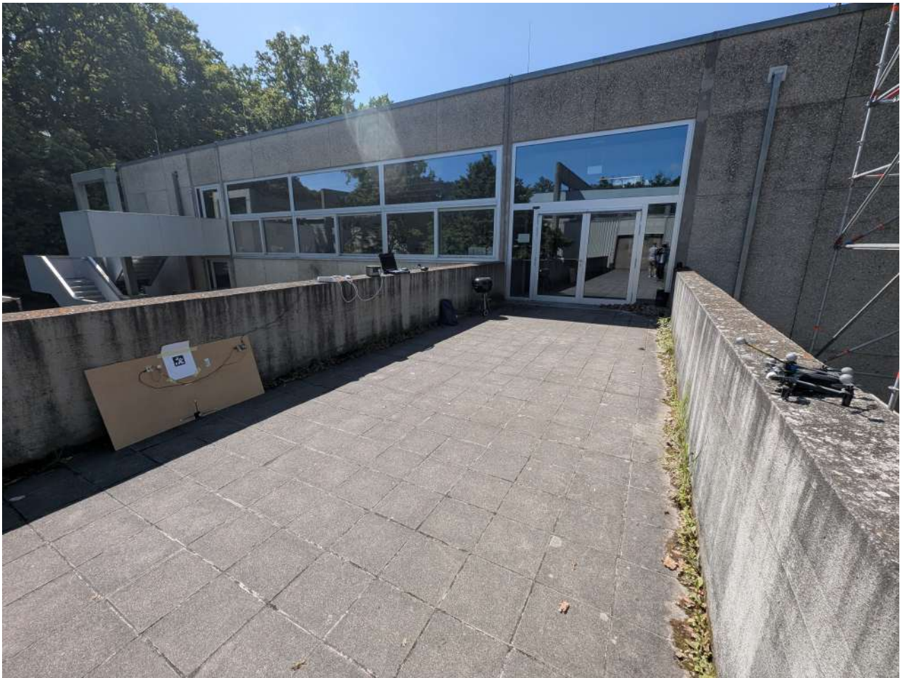
Figure 4.13: Image of setup for testing outside.
