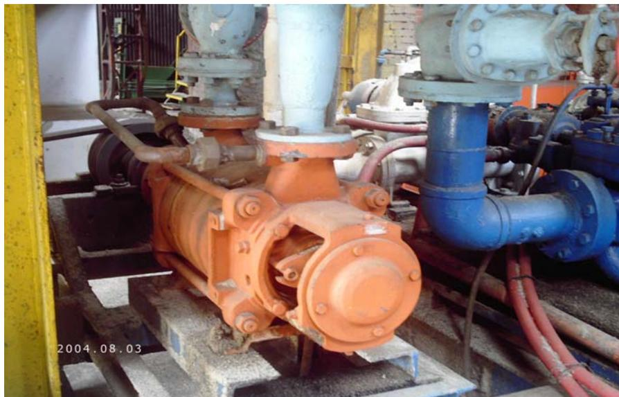
Figura C1.3 Bomba B1 Worthington 200 GPM
