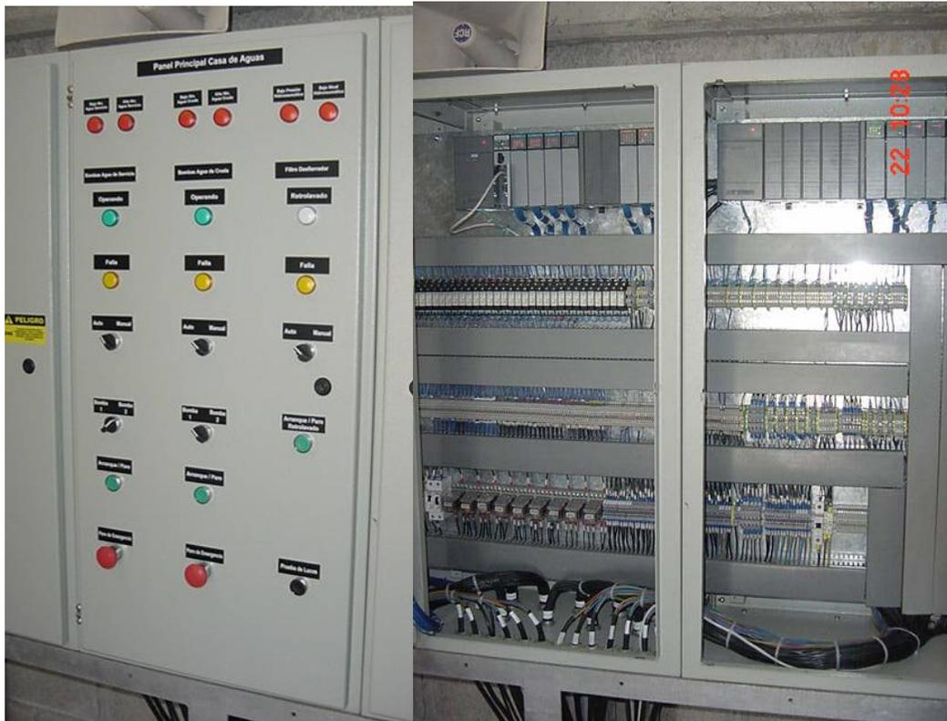
**Figura 6.5** Panel Principal y alambrado interno
