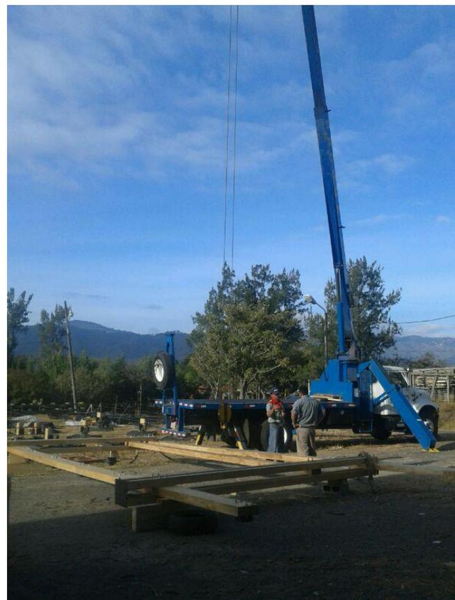
**Image 9.1.3.1.** Structural frames assembly and placing on the footings
