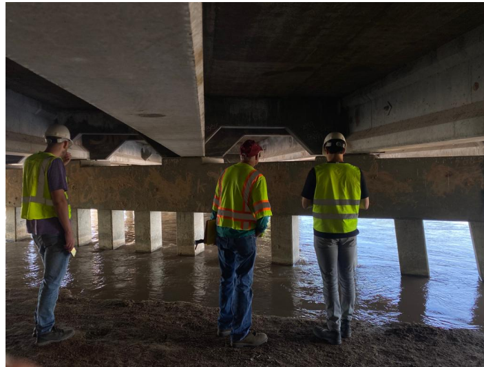
Figure 7. Team A inspecting accessible spans.
