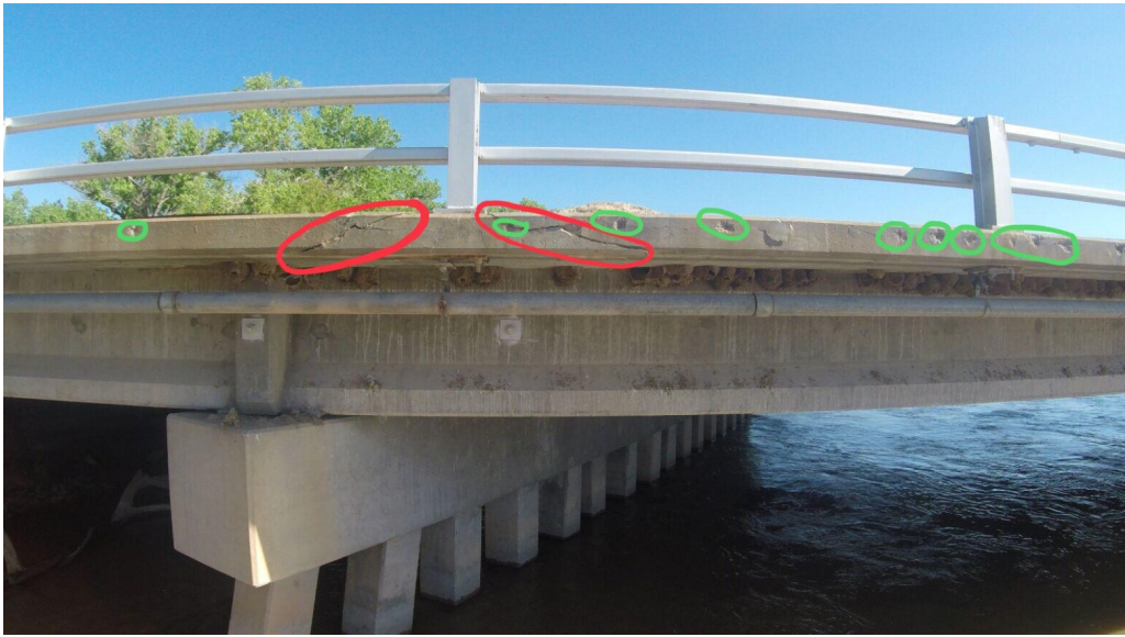
Figure 12. Cracks on deck-side and outer girder on North view.
