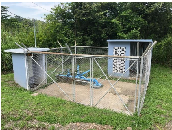
Figure 11 Pumping well 3 and chlorination station
