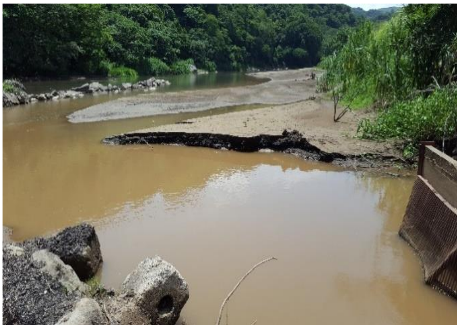
Figure 13 Surface water intake sediment
