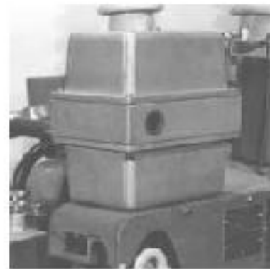
Figure 36. Remote closing solenoid.
