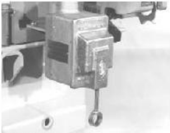
Figure 26. Ground-trip blocking switch; hookstick-operated.
