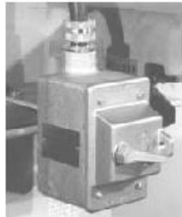
Figure 27. Ground-trip blocking switch for remote manual operation.
