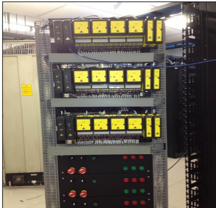
**Figura 1.** Rack de S.I.S. DeltaV Logic Solvers.
