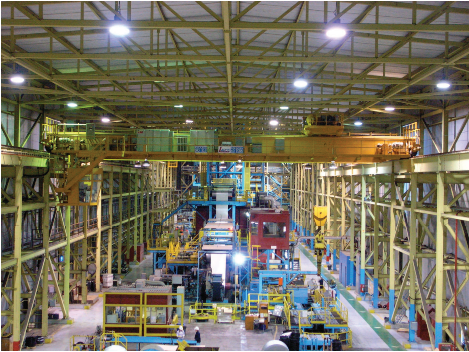
Photo 1 – Typical Laced Column Runway System
