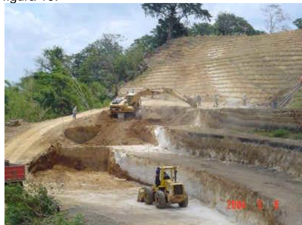
Figura 10. Talud de corte (Ref. Internet 1)
