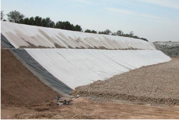
Figura 11. Talud de relleno (Ref. Internet 2)
