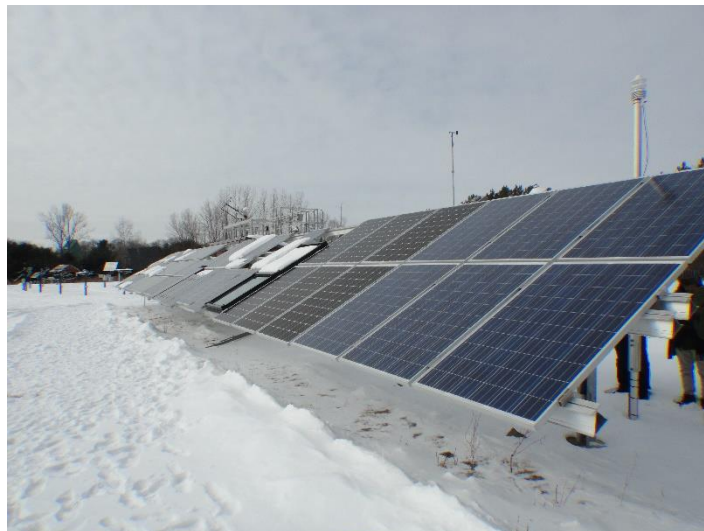
Figure 2-9 Installation of PVPV at Kortright Center.
